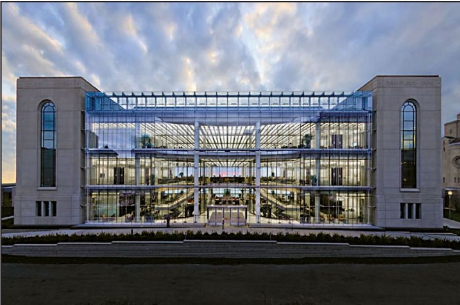
FIGURE 1. The radiant cooling system used in the ceiling at Klarchek Information Commons was designed to meet 60% of the sensible cooling load with approximately 4 W/sq ft of cooling power at 80% ceiling coverage.
