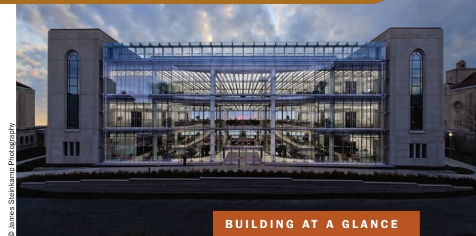
East and west glass façades preserve campus views of Lake Michigan. Masonry "bookends" on the north and south ends house classrooms.
